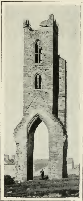
MAGDALENE STEEPLE, DROGHEDA. (Showing the damage done by Cromwell's cannon to the battlements.)
